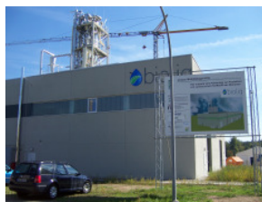
Bioliq, pyrolysis/gasification (Germany)
